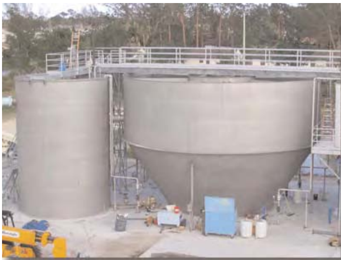
RL Pratt WTP MIEX ® Contactor & Settling Vessels
