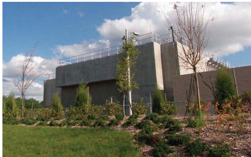
Figure 1: MIEX® System at H. Clay “Junk” Whaley, Sr. Memorial Water Plant in St. Cloud, Florida
