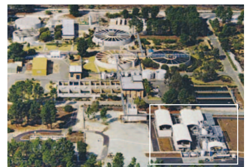
Figure 2 MIEX® Pre-treatment Plant
